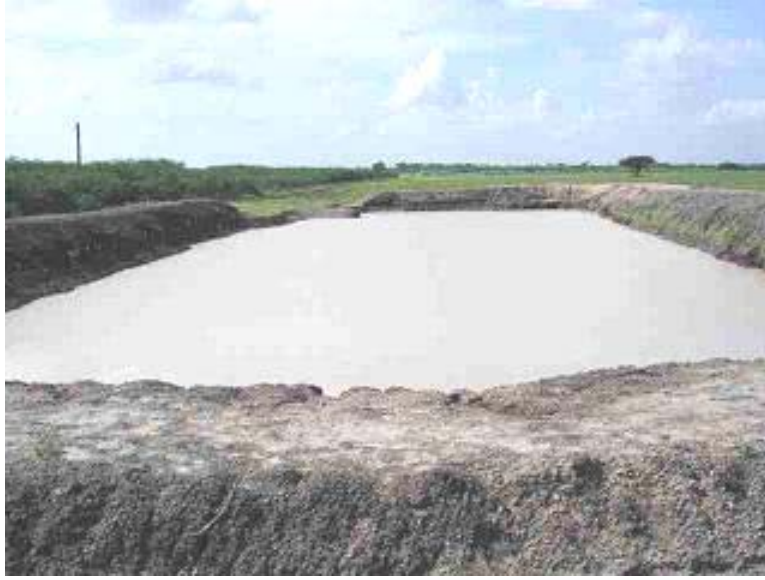
Water Harvesting Pond
